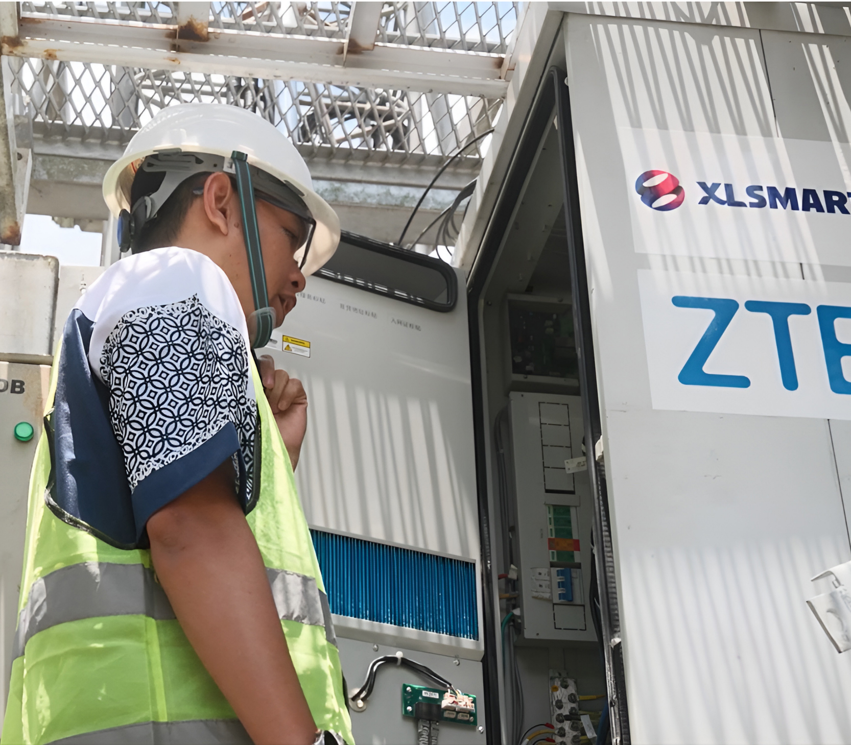
技术人员正在进行基站检测 A technician is conducting base station inspection.
